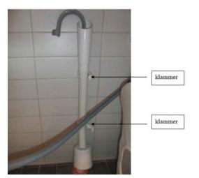
3. Disconnect the drain hose and loosen the clamps. No tools needed.
