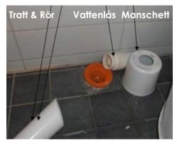
5. Remove the funnel, pipe, trap, and rubber sleeve, and clean all parts thoroughly, especially the trap.
