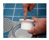
3. When putting the trap back, make sure the rubber seal fits tightly to prevent odors from escaping through the pipes.
