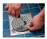
1. Remove the strainer (the metal cover).
